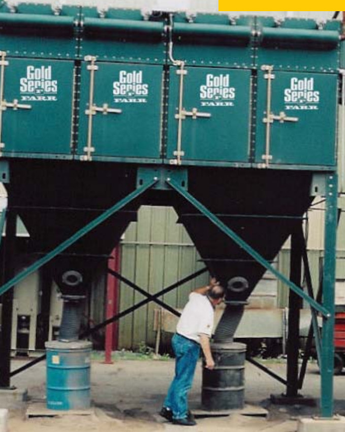
GS 48 on RR Car Sand Blasting
