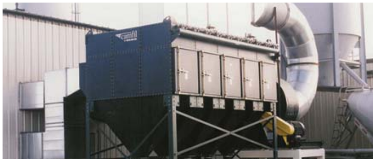
GS 60 on Sand Blasting
