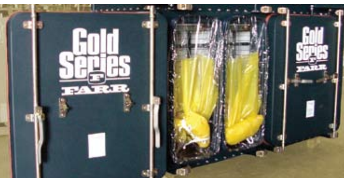
GS8 Containment Dust Collector Filter Change-out
